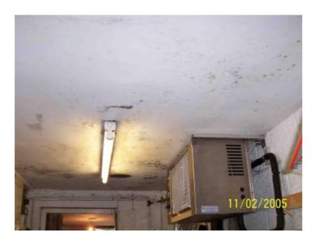
**Material** Comments: AIB suspected behind plasterboard ceiling
