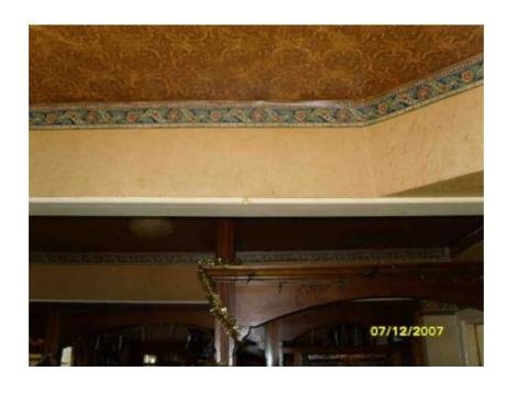
Material Comments: All structural beams may have AIB cladding beneath plasterboard exterior finish.
