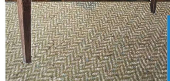
Wilton Carpet abutting dark stained timber plank
